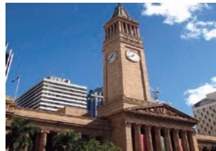
Brisbane City Hall, QLD Consultant EMF Griffiths Installation Siganto and Stacey ACDHUM2-W & ACDHUM3-W
