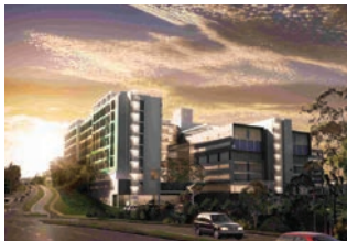
Gold Coast University Hospital, QLD Consultant SKM Installation Hastie Air Conditioning 13 various ACDHUM6-W, ACDHUM7-W & ACDHUM8-W
